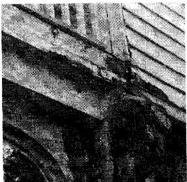
Due to the dilapidated siding, water damage was accumulating inside the house.
