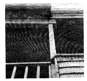
Parts of the siding and soffits were missing, exposing the plywood underneath.
