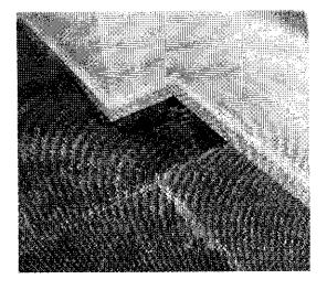
For the replacement siding, we chose a color (Navajo Beige) similar to the existing color. The material, fiber cement siding (Hardie Board), is an upgrade from the existing material. The replacement soffits and eaves are white, the same color as the old soffits and eaves.
