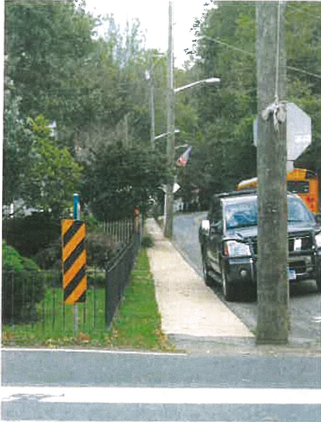
PLATE 4 View from Main St. and School St., Looking South
