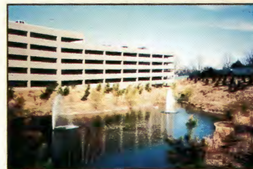
Stormwater ponds protect water quality by slowing and filtering runoff from developed areas.
