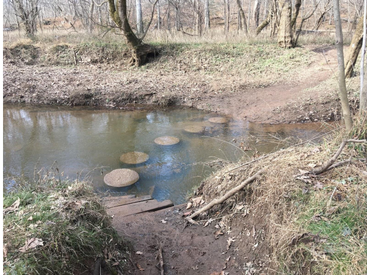
Bull Run-Occoquan Trail concrete pillar crossing Little Rocky Run in high water stage 13
